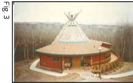
Figure 3: Healing Lodge (meeting and ceremonial area) at Okimaw Ohci, Photograph: Correctional Service, Canada. The basis of the design of the lodge is the Nekaneet First Nation's tipi ethno architectural tradition and the medicine wheel. The master plan for the facility and individual buildings are circular (with minor adjustments for functionality). The facility is located near the sacred Thunder Hills of southwest Saskatchewan.
