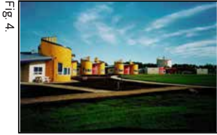
Figure 4: Pê Sâkâstêw Centre, Alberta. Photograph: Correctional Service, Canada. The Centre was designed consultation with Samson Cree Elders. The architecture symbolises the Aboriginal view of the world, with each of the six yellow buildings a tall, conical shape and the group arranged in a large circle on the 40-acre site. Bright primary colours herald Aboriginal ancestry, as does the eagle tail entrance to the main programming building.
