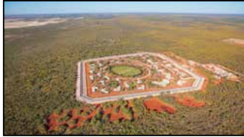
Figure 7: West Kimberley Regional Prison, Western Australia. Photograph: Peter Bennetts. West Kimberley Regional Prison is designed to house male and female prisoners in self-care units. The 22 houses on site accommodate 6 to 7 prisoners each and are grouped so that prisoners can be located according to family ties, language and security rating.
