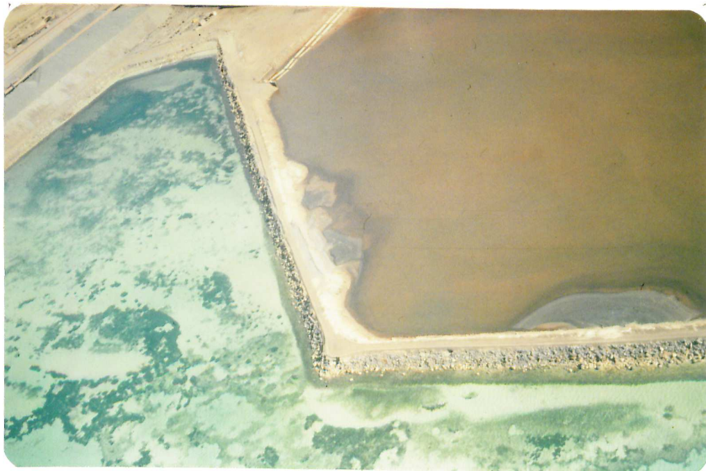
PLATE 3.1 Tailings dam wall.
