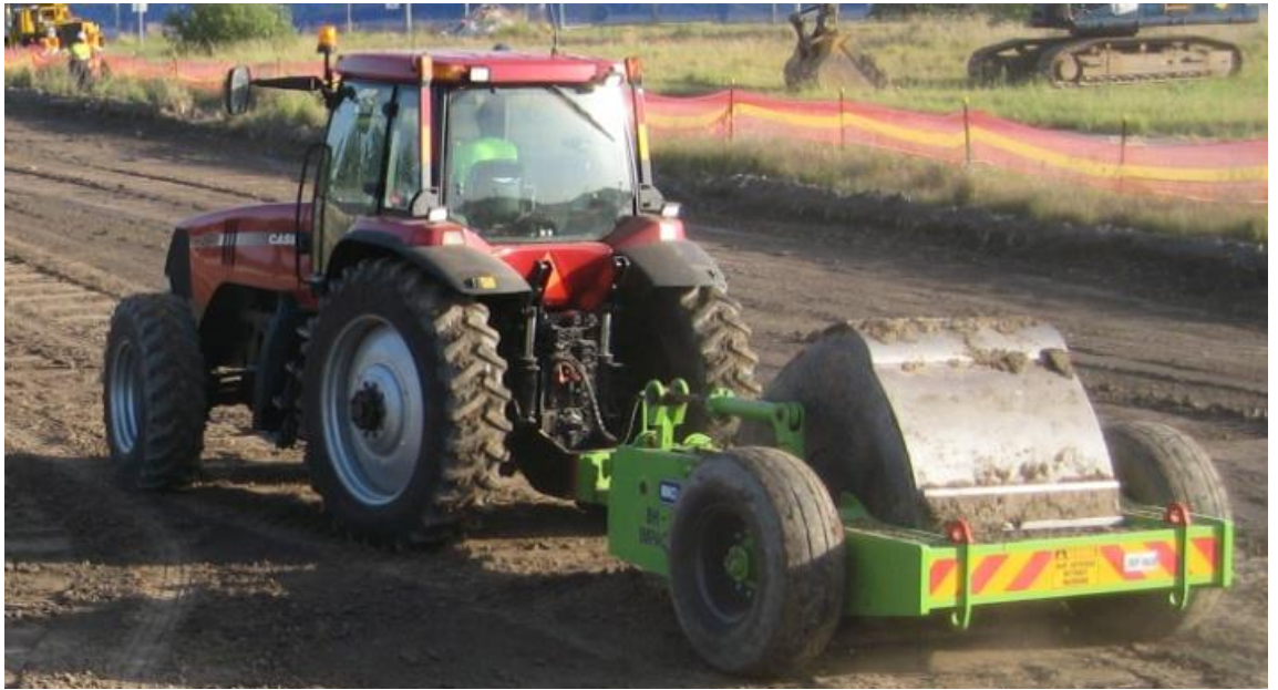
Figure 2. Impact rolling in progress.
