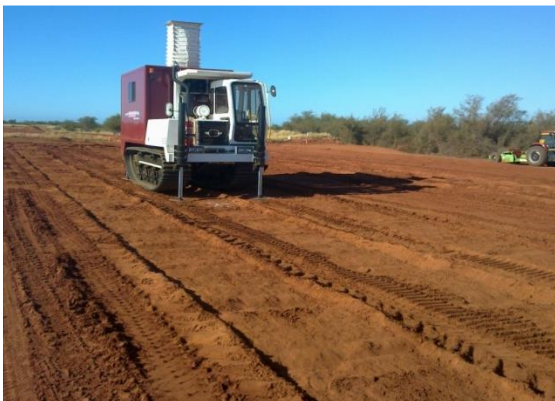
Figure 2. CPT rig undertaking post compaction testing
