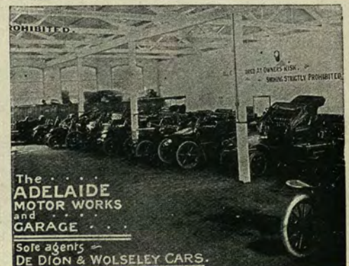
Interior of Garage
