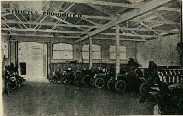
Interior of Garage.
