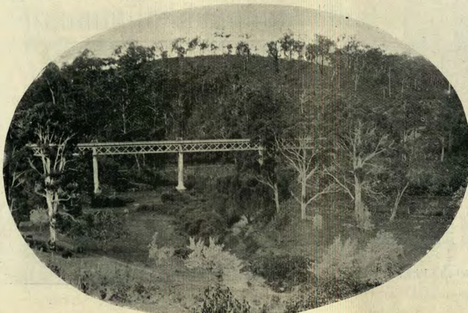
Railway Bridge at Bridgewater
