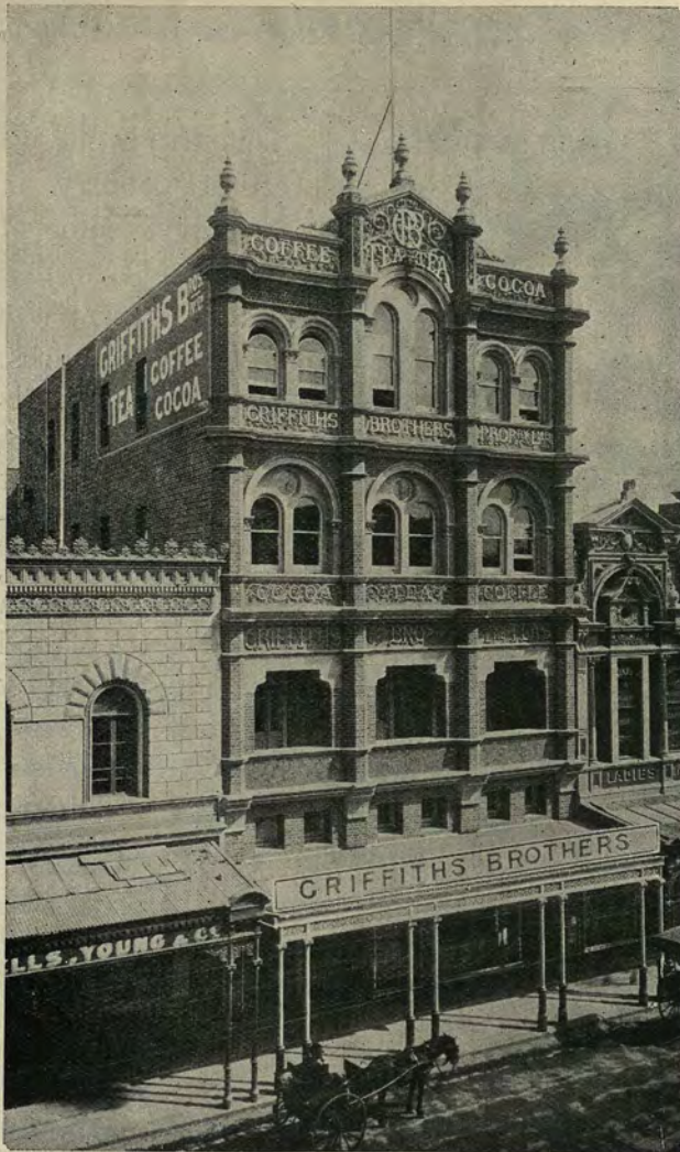
View of Warehouse.
